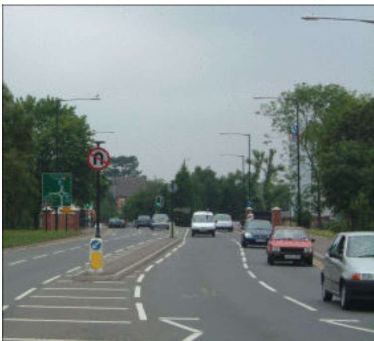
Picture 3.1 Nuneaton Ring Road
