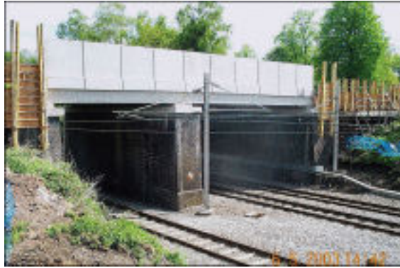
Picture 3.7 Bridge maintenance in progress near Brinklow
