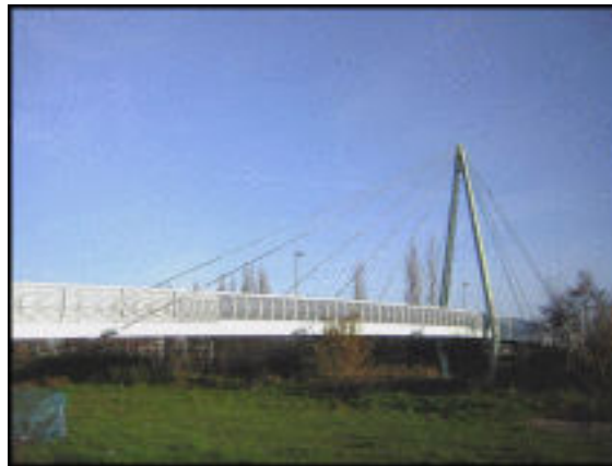
Picture 3.3 Maple Park Footbridge
