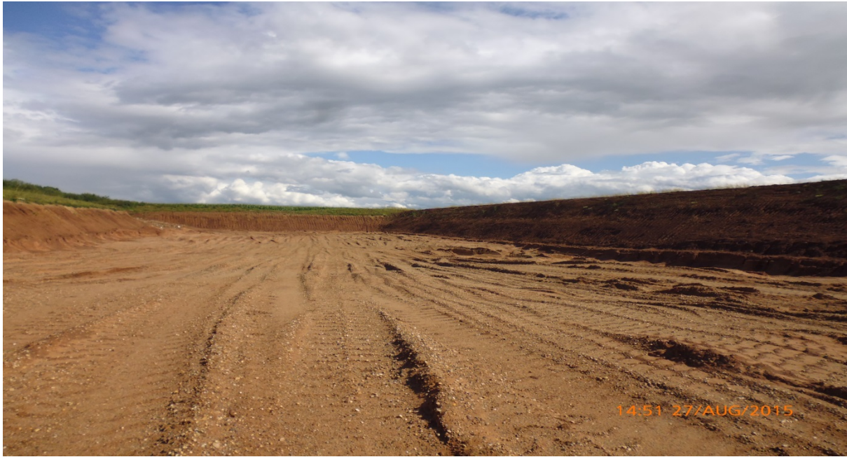
Fig 3 Excavation of sand and gravel beneath overburden at Brinklow Quarry
