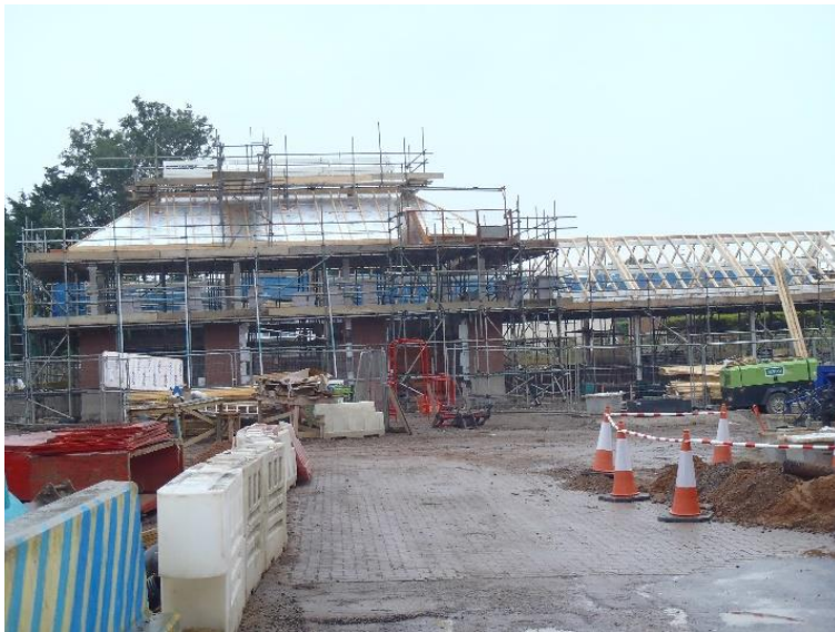
The New Station September 2017
