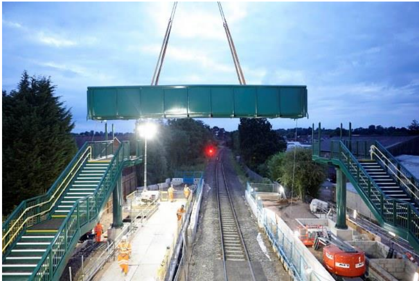
Bridge Lift July 2017
