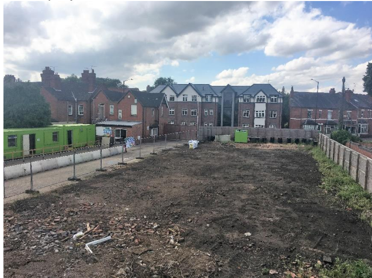
Clearing the Site 2016
