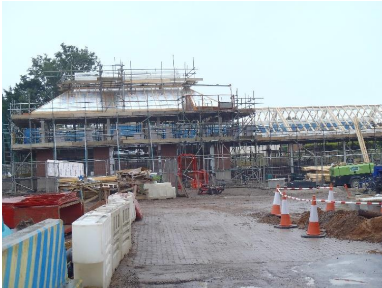
The New Station September 2017
