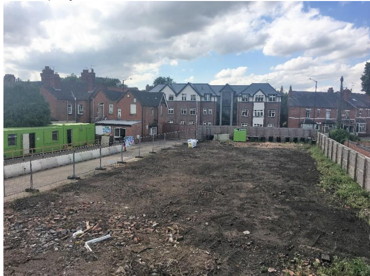
Clearing the Site 2016
